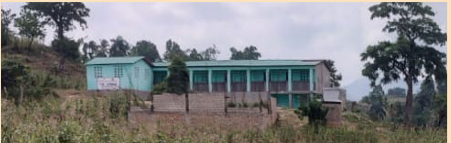
This is the building where the Satellite Trade School will hold classes for the first year.
