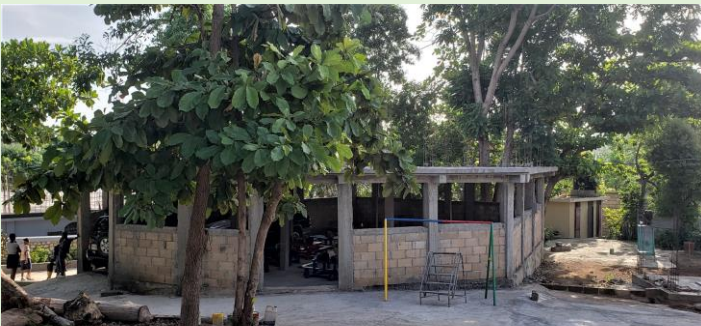
The exterior of the completed Gathering Center. What a huge praise to our Lord!
